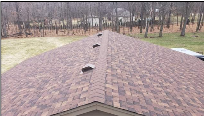
"Walk On Roof" Inspections Performed
