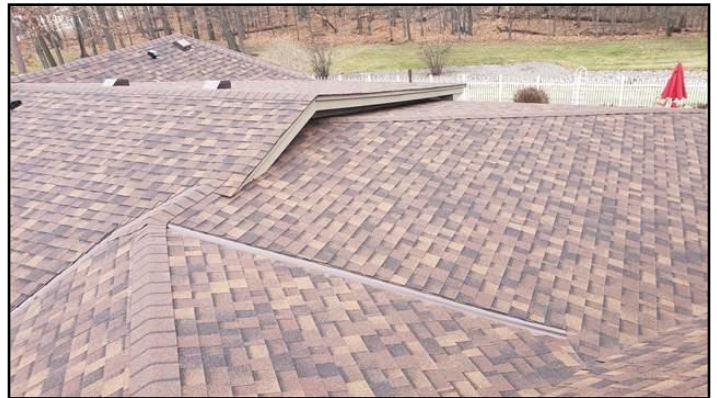
"Walk On Roof" Inspections Performed
