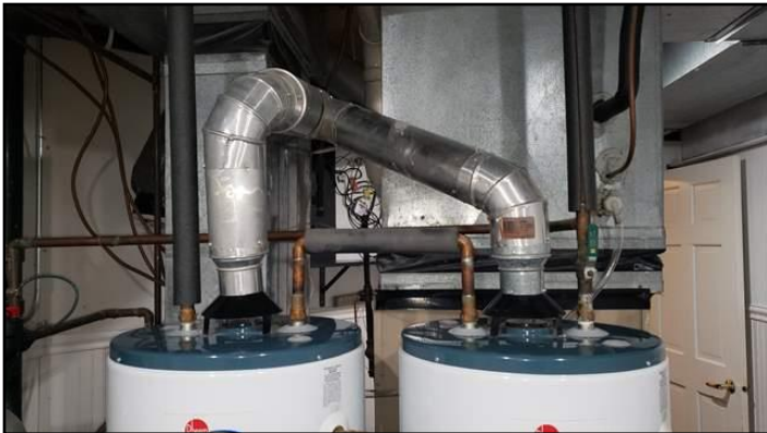
Exhaust Vents & Water Pipes Inspected
