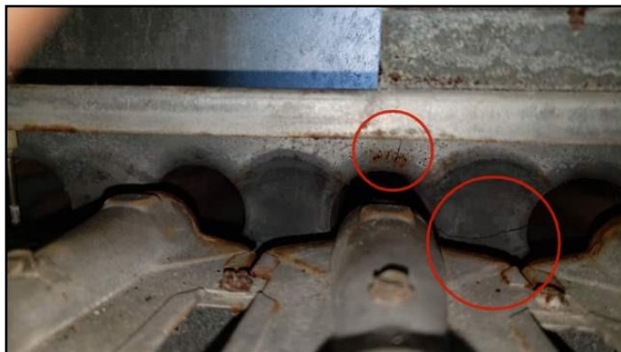
Cracked Burners
