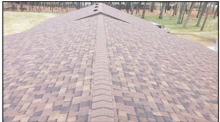
"Walk On Roof" Inspections Performed
