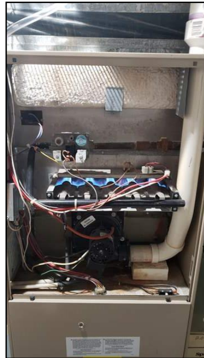
Furnace Cabinet Inspected
