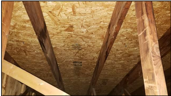
OSB Sheathing Inspected
