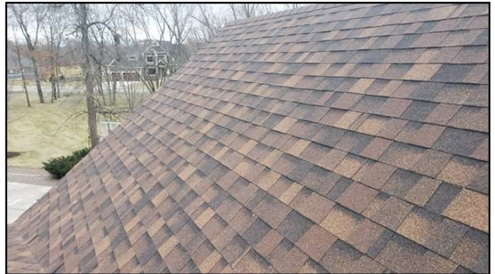
"Walk On Roof" Inspections Performed
