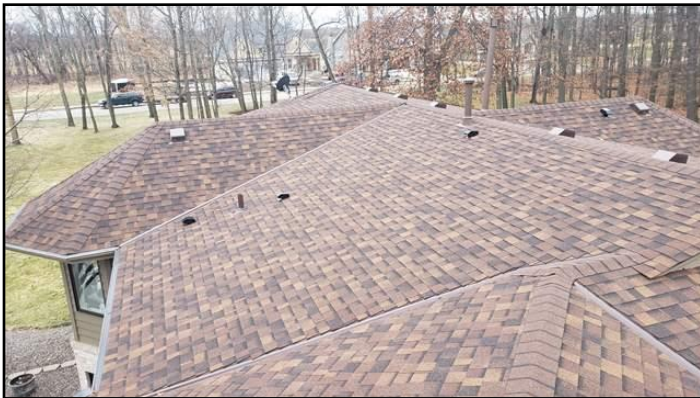
"Walk On Roof" Inspections Performed
