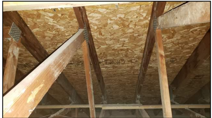
OSB Sheathing Inspected
