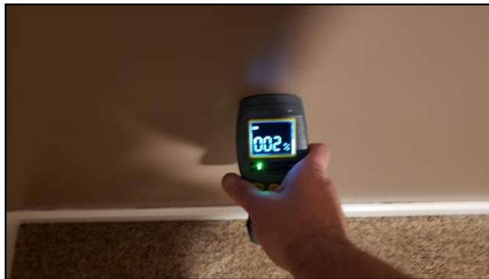
Wall Moisture Test Performed
