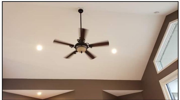
Ceiling Fans Ran and Functioning
