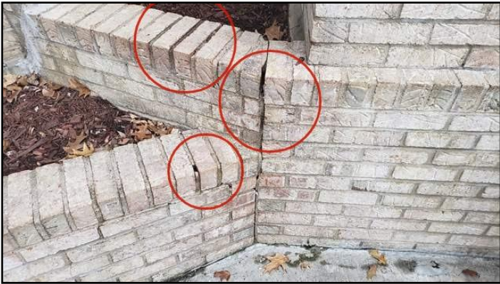
Deteriorated Mortar
