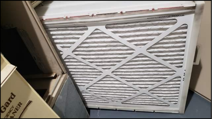
Furnace Filter Inspected
