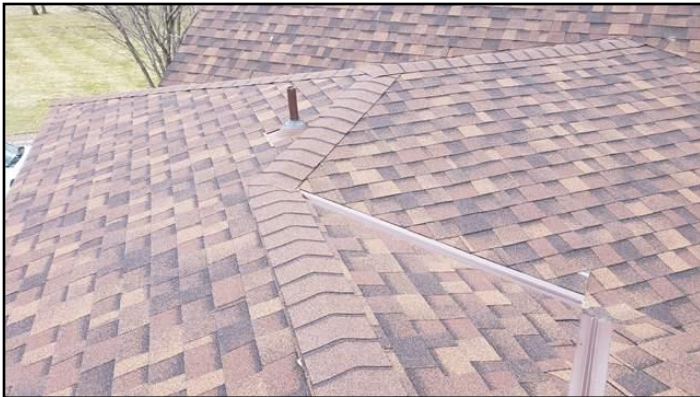
"Walk On Roof" Inspections Performed
