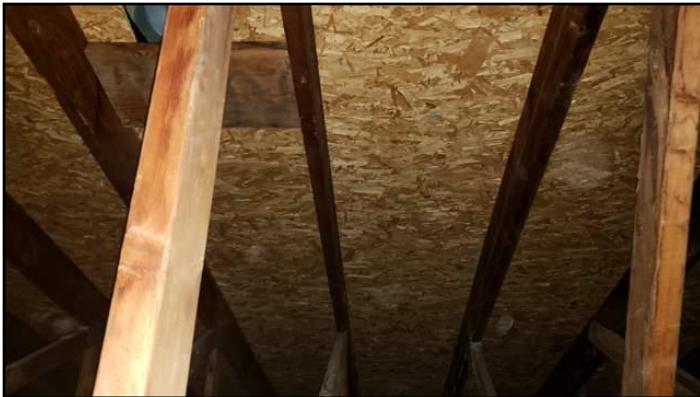
OSB Sheathing Inspected
