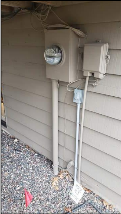
Service Entrance Inspected
