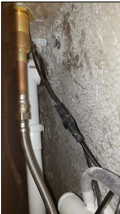
Tub Overflow Tested For Leaks
